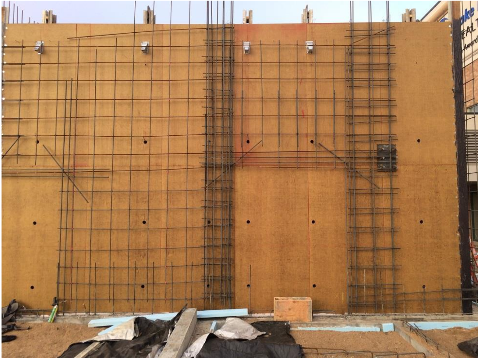
Rebar tied for first level of Stair B location with door openngs.
