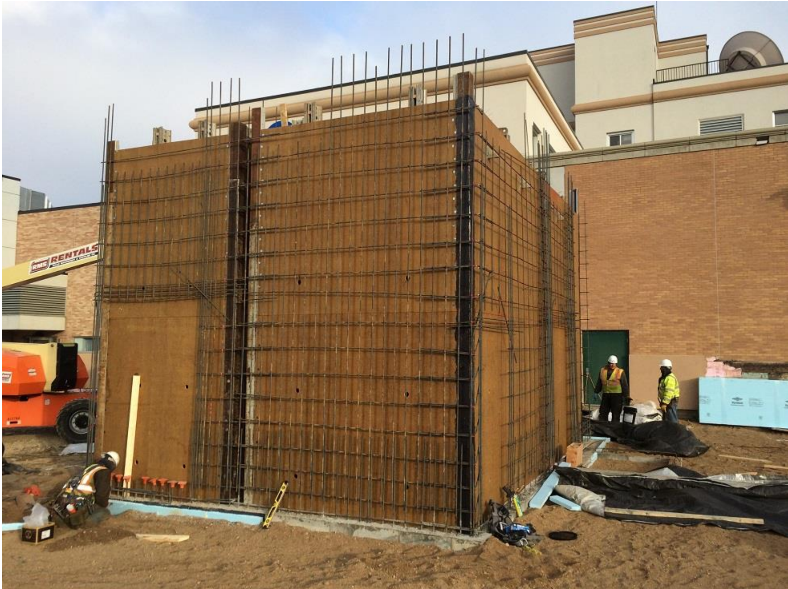
Stair B core walls being formed.
