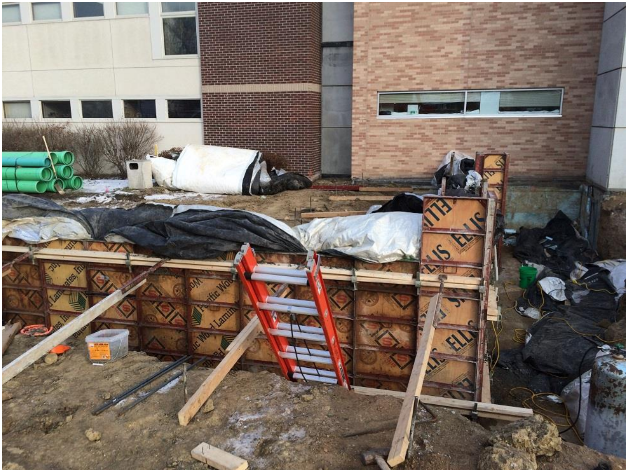
Foundation grade beams poured on the north side of building.
